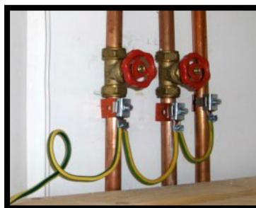
Older houses often have bonding wires of 6mm<sup>2</sup>, 4mm<sup>2</sup>, 2 mm<sup>2</sup> or even no bonding at all.
