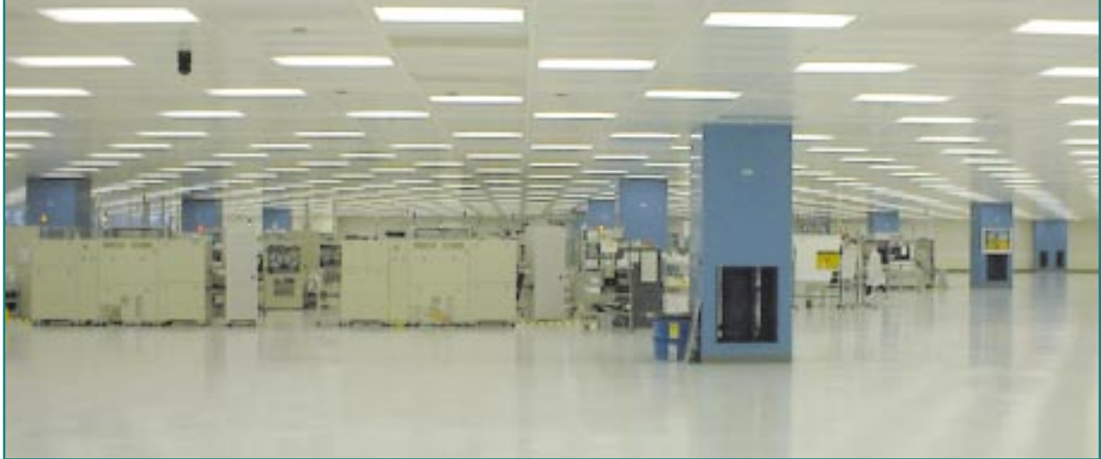
Cleanrooms at Hewlett – Packard.
