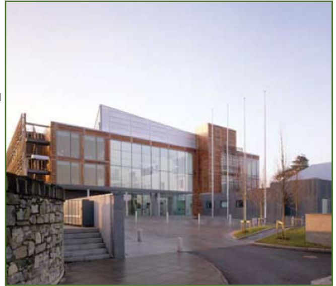
Offaly County Council's Aras an Chontae has won Best Sustainable Building 2003 awards from An Taisce and the Royal Institute of Architects of Ireland for its headquarter building incorporating ground source heating.
