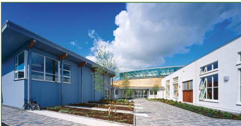
Gaelscoil An Eiscir Riada, Tullamore. First low-energy school in Ireland (Photography - Gerry O’Leary)
