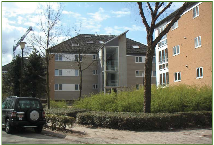
Renovated apartment block for social housing in Vorselaar, Belgium. The roof of the central staircase supports the solar water heating panels
