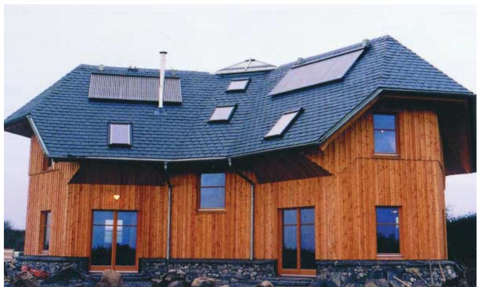
Thermomax's Award-winning evacuated tubes on a new timberframe house in Ireland
