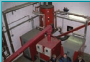
Inside the boiler house
