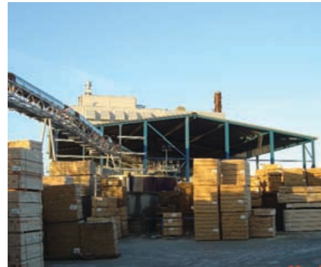
Construction of the covered fuel conveying system
