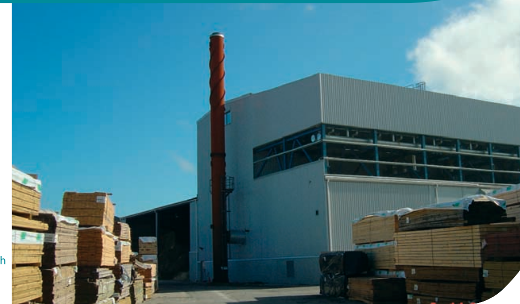
Grainger's Sawmill CHP Plant
