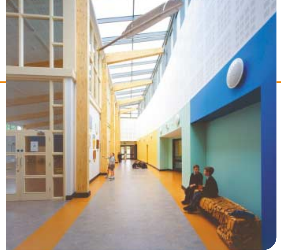
High level atrium encourages natural ventilation and provides natural light deep into the building
