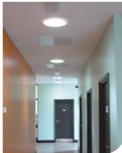
Sun pipes provide natural light in corridors
