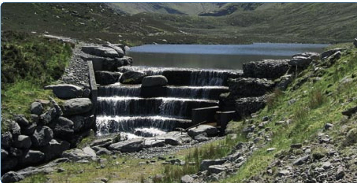
Barrier without fish pass on outflow of impounded lake.
