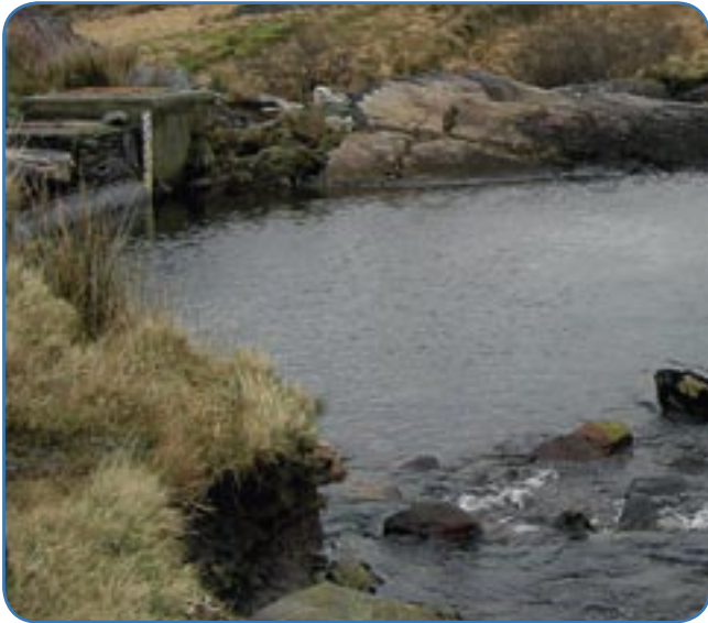
Two examples of a natural rock head weir downstream of intake on a high head run of the river scheme.
