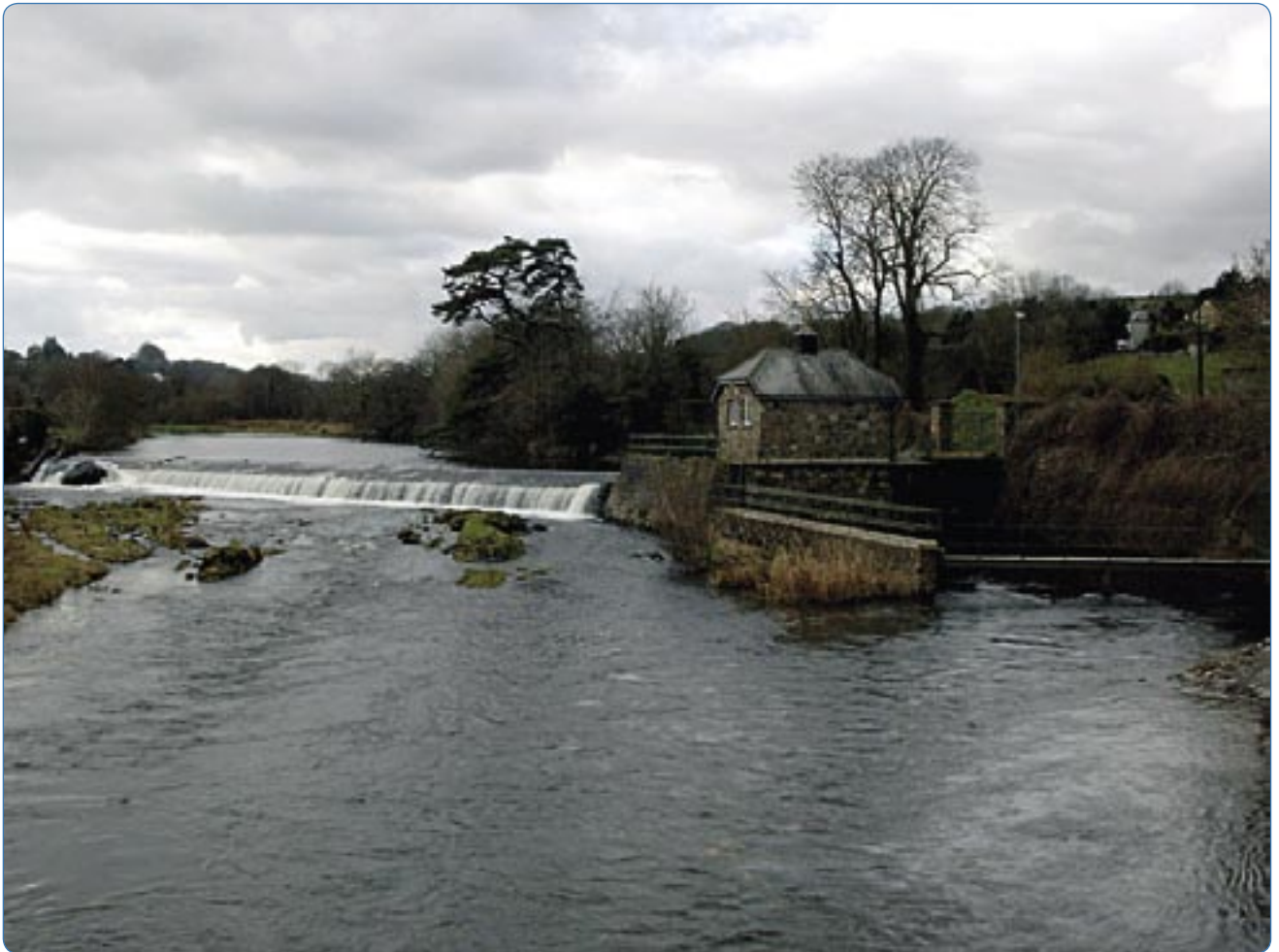
Low head hydro scheme on the Bandon River. The intake is located above the weir (right background) and the tailrace discharges back to the main river (right foreground).
