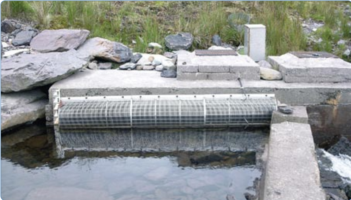
Intake screen arrangement at a high-head site.
