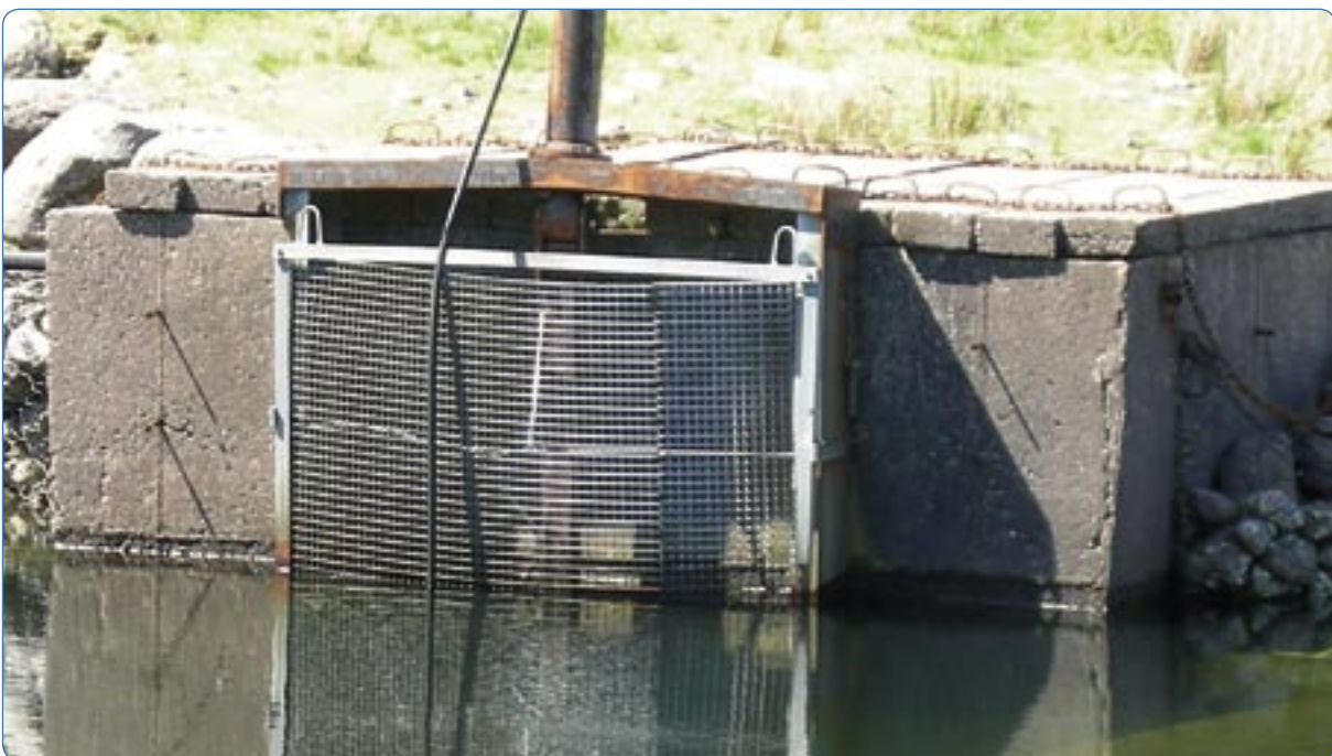
High head run-of-river intake screen.
