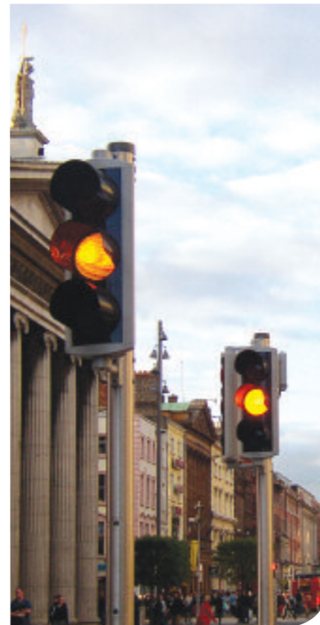
Updated traffic signals at O'Connell Street
