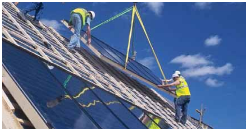
Installation of Solar Panels at Inchydoney Island Lodge & Spa.
