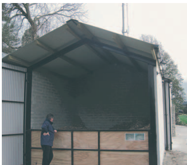
Wood chip storage at Brook Hall
